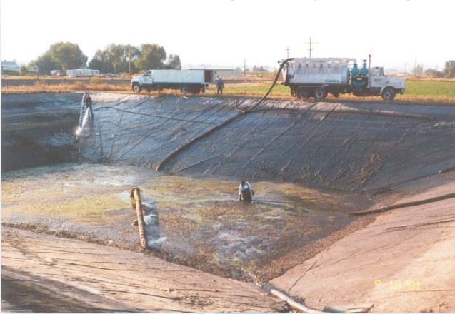
Sludge Removal from Existing Pond
