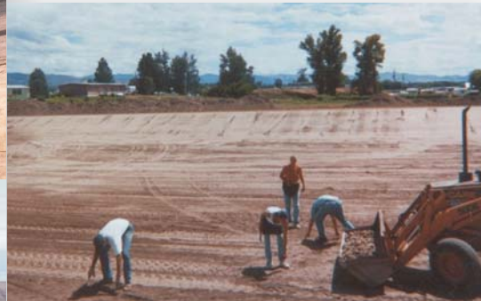
Hand Picking Rock, Prior to Liner Installation
