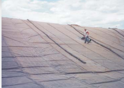
(Exposed) Liner Seaming/Ballast Tubes
